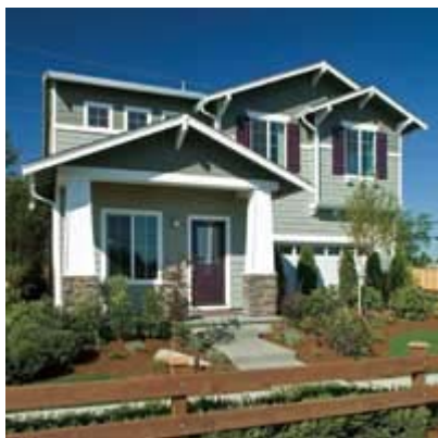
Courtesy Centex Homes HEAD EAST YOUNG HOME BUYERS: Houses in Centex Homes' East Pointe community in Kent, Wash., range in size from 1,513 to 2,801 square feet with base pricing from $349,000 to $439,000.
